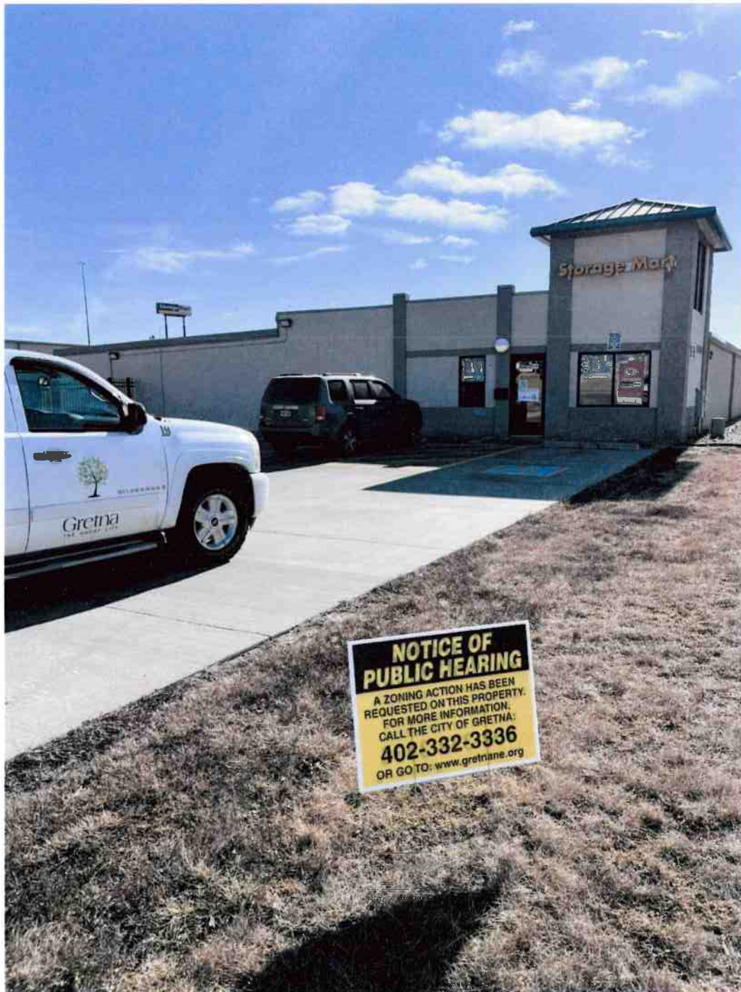
Lot 1, 370 STORAGE (11001 Sapp Brothers Drive) facing East.
