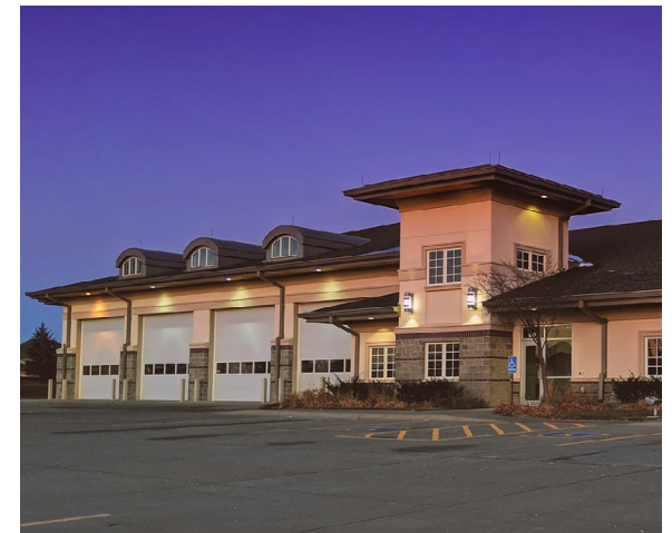
Gretna Fire & Rescue, Station 2 10309 S. 168th St
