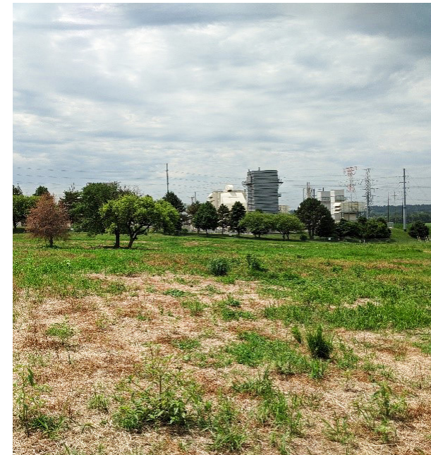
Sarpy County Peaking Station Combustion Turbines
